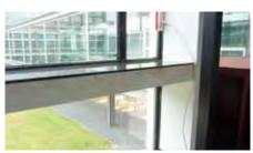
Figure II.1.93: water infiltration at windowsill.
