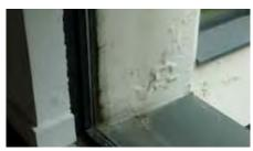
Figure II.1.98: bubble formation coating.
