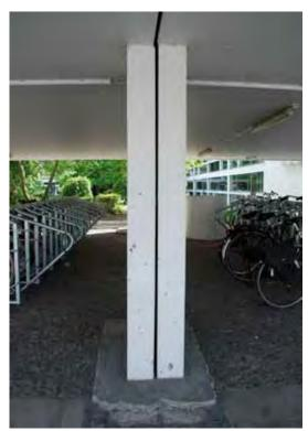
Figure II.1.2: Acoustic joint: deduplicated columns (MH, 23/05/2014).
