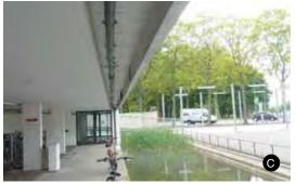
Figure II.1.9: Horizontal rainwater downpipe (note: the finishing panel is missing).
