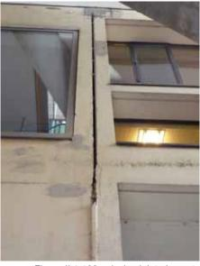
Figure II.1.100: missing joint element.
