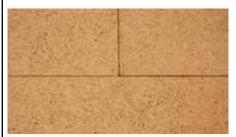
Figure II.1.44: woodwool cement ceiling.
