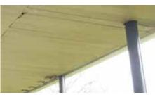
Figure II.1.91: deformations lamella.
