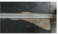
Figure II.1.87: damaged corner linoleum.
