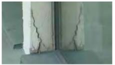
Figure II.1.96: cracks due to concrete degradation.
