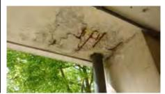
Figure II.1.97: uncovered concrete.
