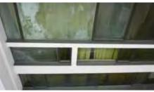
Figure II.1.103: internal condensation glass.
