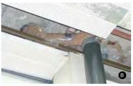
Figure II.1.8: connection rainwater downpipe.
